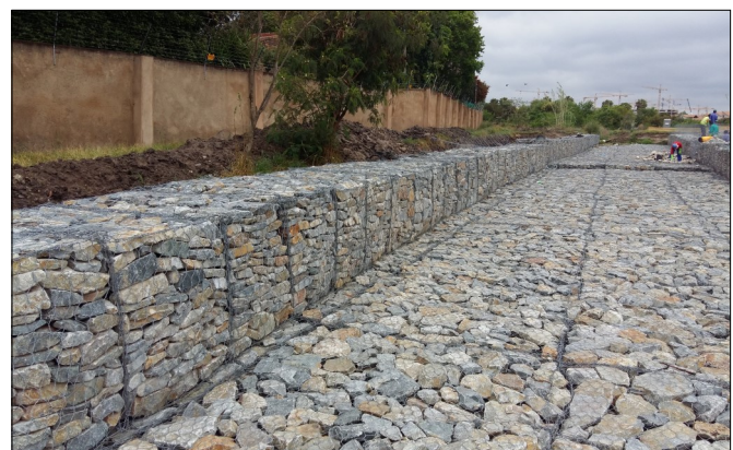
Figure 3: Gabion Zinc & Polymer coated
